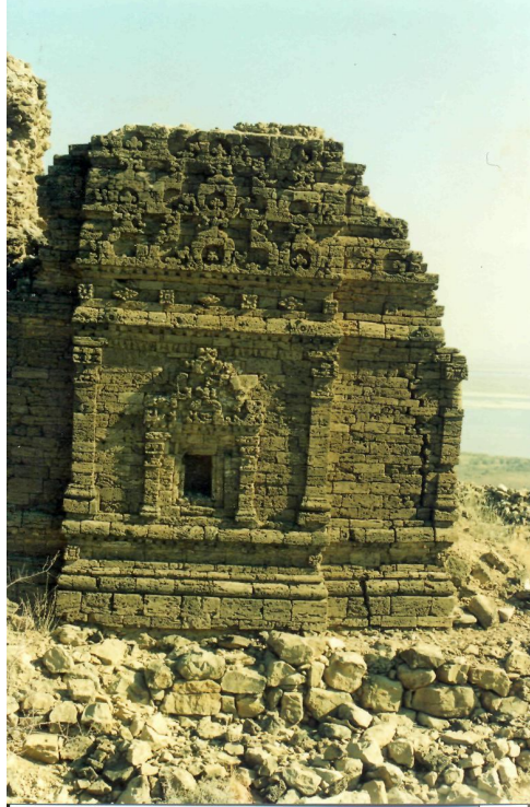
North Kafir Kot: Temple C. Details of the western wall
